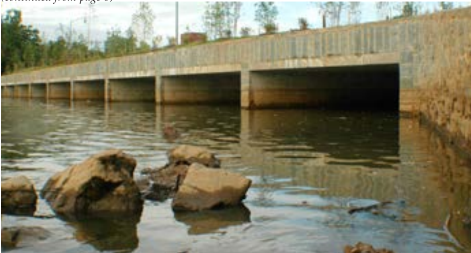
Whitman, Requardt & Associates, LLP Division C - CSO 019 Overflow and Diversion Structures
