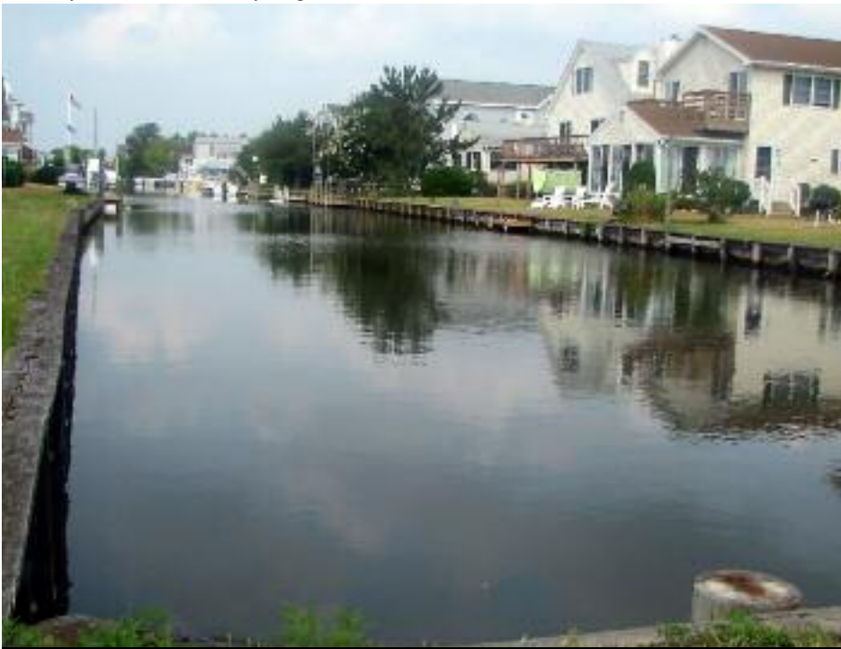
2008 GRAND AWARD and OUTSTANDING PROJECT IN GROUP 1: Studies, Research and Consulting Engineering Services - South Bethany Tidal Pump System (DE) - KCI Technologies
