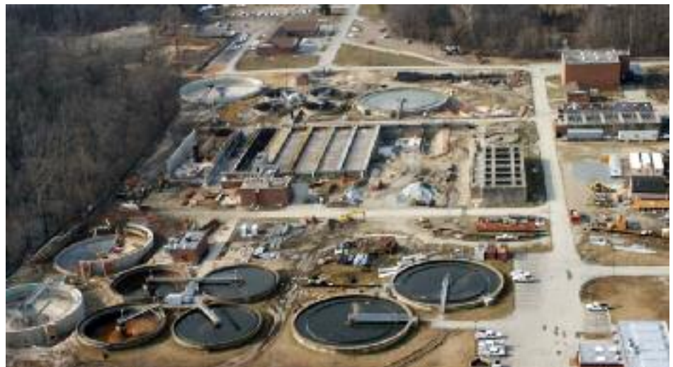
OUTSTANDING PROJECT IN ENVIRONMENTAL - Mattawoman Wastewater Treatment Plant – Joint Venture – George, Miles & Buhr / KCI Technologies
